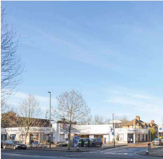
The existing station entrance is not apparent, even when the trees are bare
